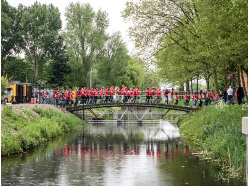
Figure 4. Test loading the Glass Truss Bridge
