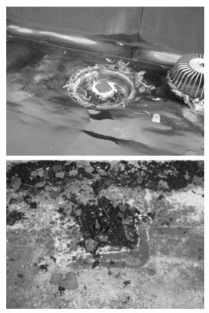
Figure 2: Examples of blocked rainwater gullies
