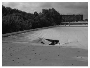
Figure 1: Example of a roof after a local collapse due to ponding
