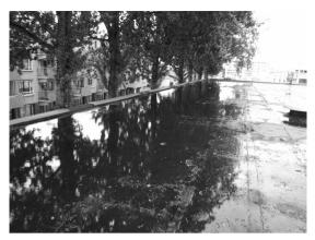
Figure 2: Rainwater ponding, no emergency overflow in the roof up stands
