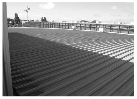
Figure 6: An example of light-weight flat roof where already the detailing only (elevated trough roof sheeting under sufficient slope in combination with lower positioned roof gutters) prevents any form of rainwater ponding that could impair the structural safety and quality of the roof
