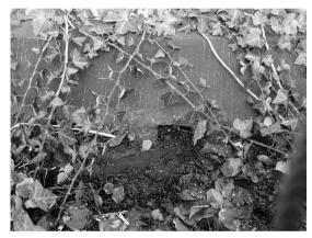
Figure 3: Plant growth and fallen leafs on the roof
