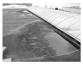
Figure 4: Light street blocking the roof slope results in ponding
