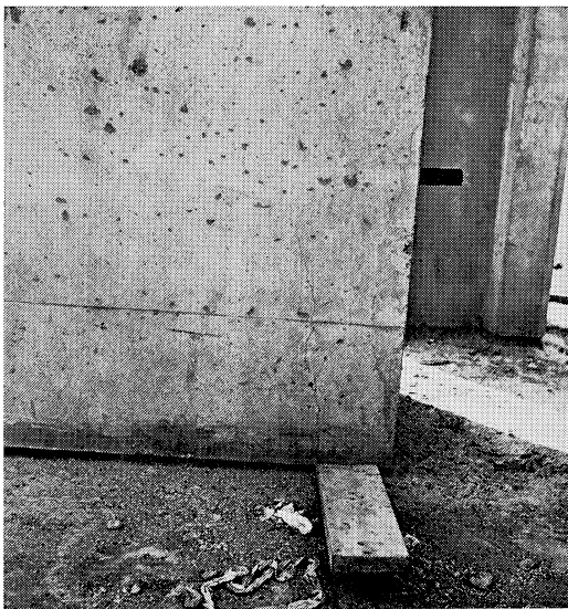
Fig. 28 Typical cracking at the end of a beam.
