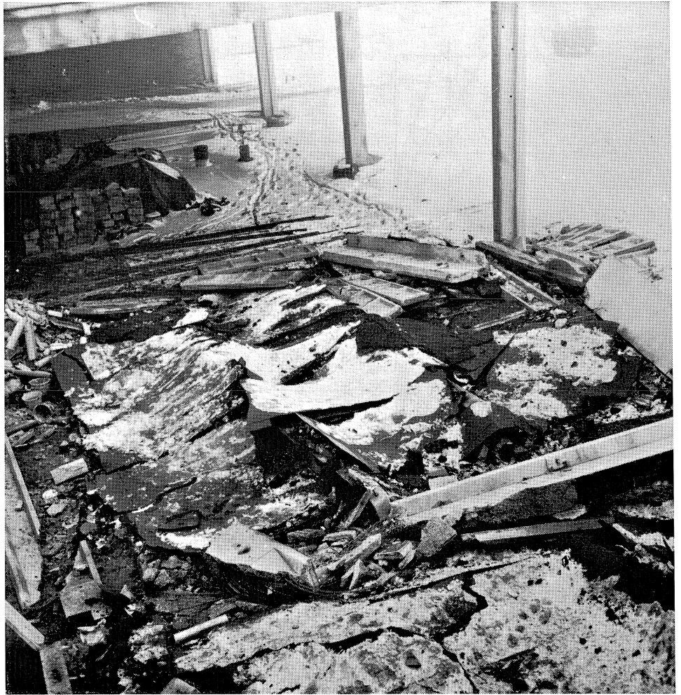
Fig. 2. Damage caused by absence of stirrup reinforcement in beams loaded through corbels (1963).
