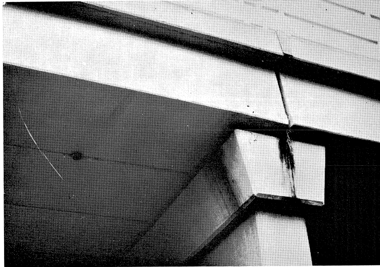
Fig. 41. Inadequate provision for rainwater discharge produced this unsightly appearance.
