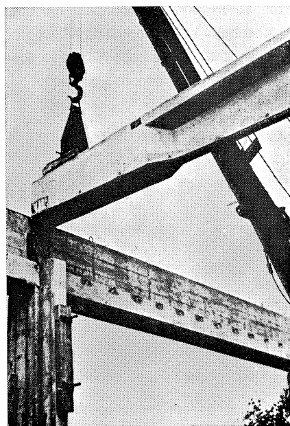
Fig. 86. Special attachment to raise the level of the slinging point and thus prevent toppling.
