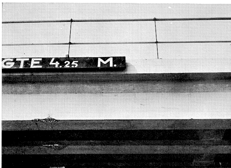
Fig. 80. Damage due to collision on a bridge con- structed from precast pre- stressed concrete beams.
