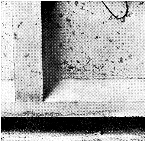
Fig. 62. Cracking due to secondary tensile stresses caused by a displaced cable duct.
