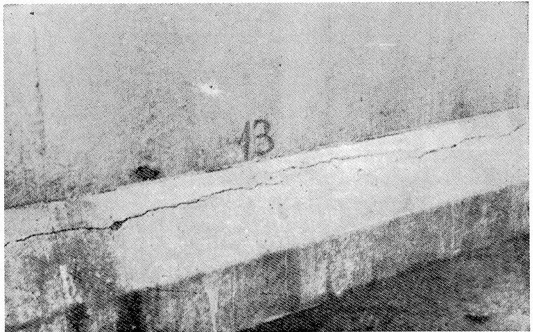
Fig. 72. Cracking due to freezing of water in a cable duct.
