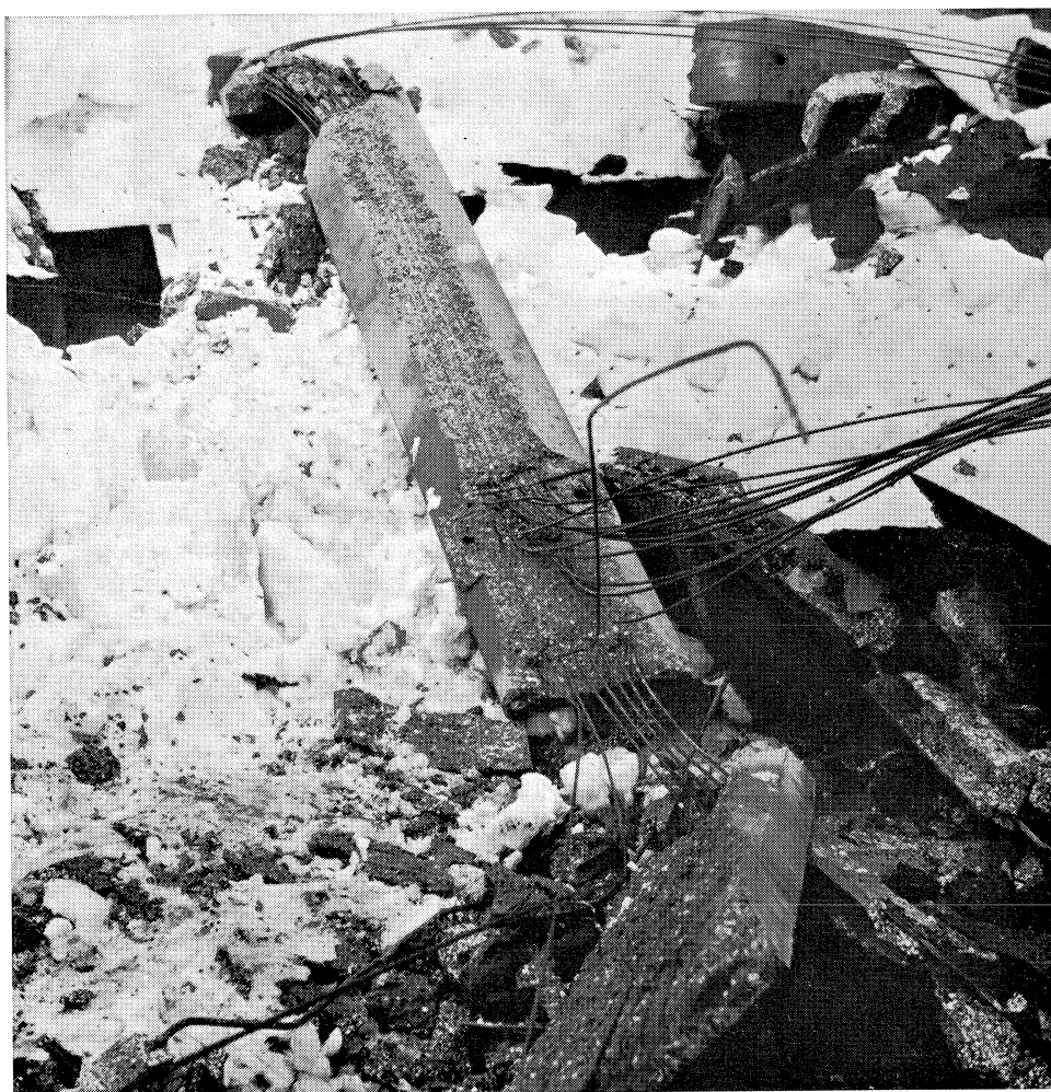
Fig. 5. Detached bottom flange of a beam loaded through corbels and containing no stirrups.
